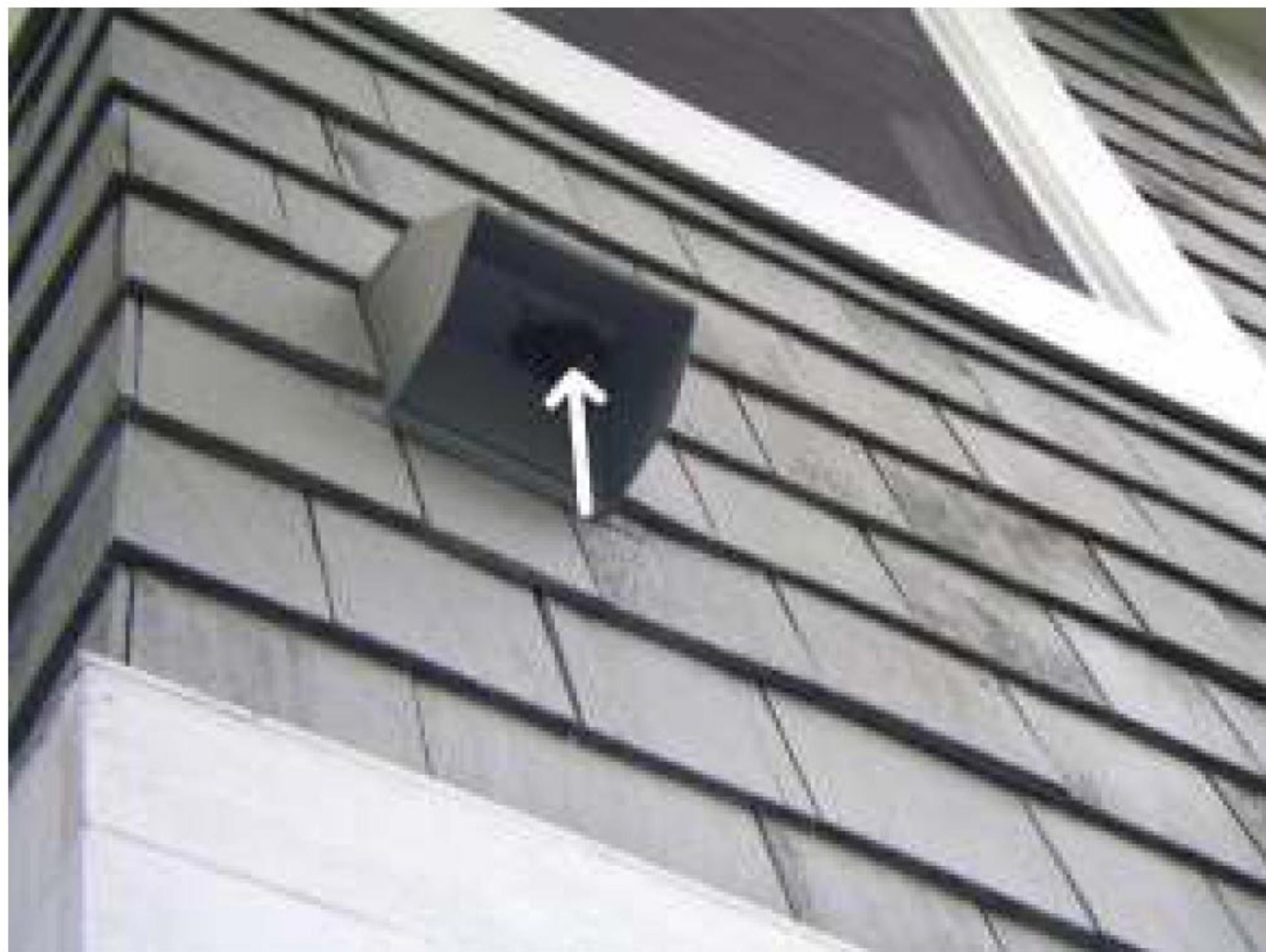
Arrow shows wasp nest at kitchen exhaust hood. Remove this fall when inactive.
